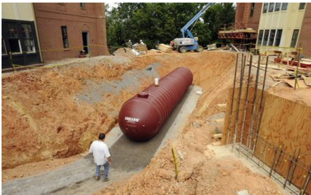
The underground rainwater cistern collects roof runoff for landscape watering.
