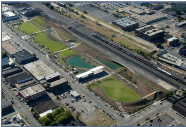
THE RAILROAD RESERVATION PARK STORMWATER SYSTEM
