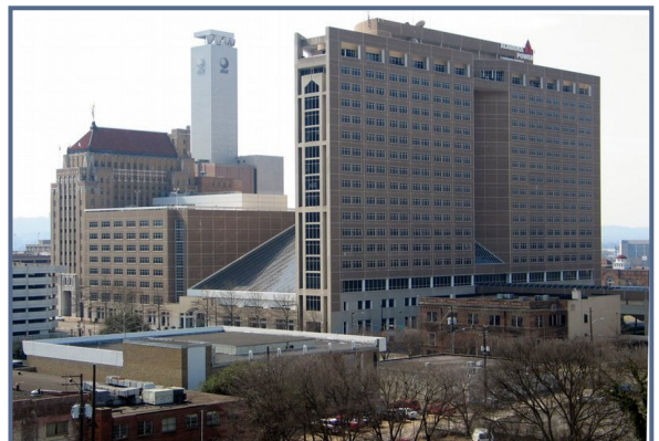
ALABAMA POWER COMPANY WATER EFFICIENCY RETROFIT
