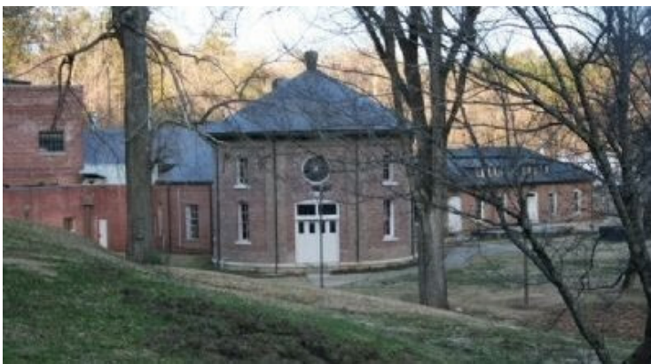
Cahaba Heights Pump Station on the Cahaba River.
